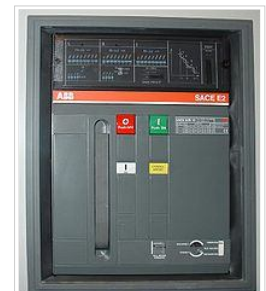
Front panel of a 1250 A air circuit breaker manufactured by ABB. This low voltage power circuit breaker can be withdrawn from its housing for servicing. Trip characteristics are configurable via DIP switches on the front panel.
