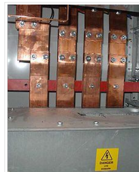
Busbars may be needed in situations requiring adequate ground conductors.
