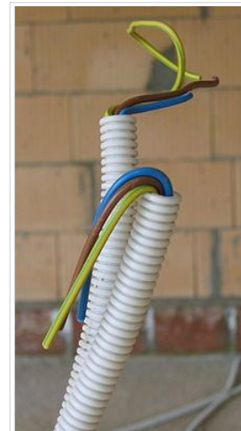
An electrical "3G" power cable found commonly in modern European houses. The cable consists of 3 wires (2 wires + 1 grounding in case if cable has "3G" name) and is double-insulated.
