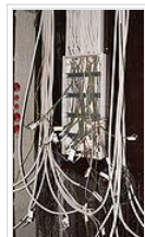
a distribution board being installed
